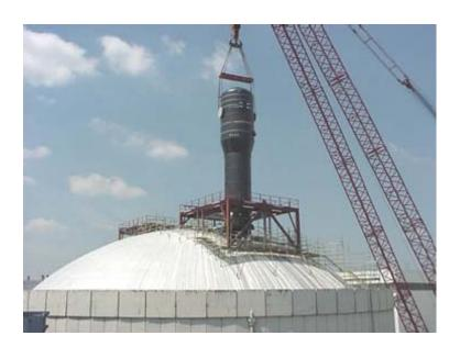
In order to remove the existing steam generators and install new steam generators, it was necessary to make two holes in the primary steel containment and in the dome of the secondary concrete containment. The holes in the primary containment had a diameter of 5.5 m, the steel being 25 mm thick. The square holes in the secondary containment had a side of 5.5 m, the concrete being 80 cm thick.
