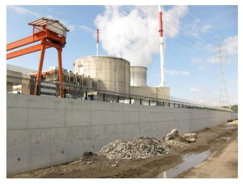
Figure 1 : Peripheral protection of the site of Tihange against beyond-design flooding realized in 2015
