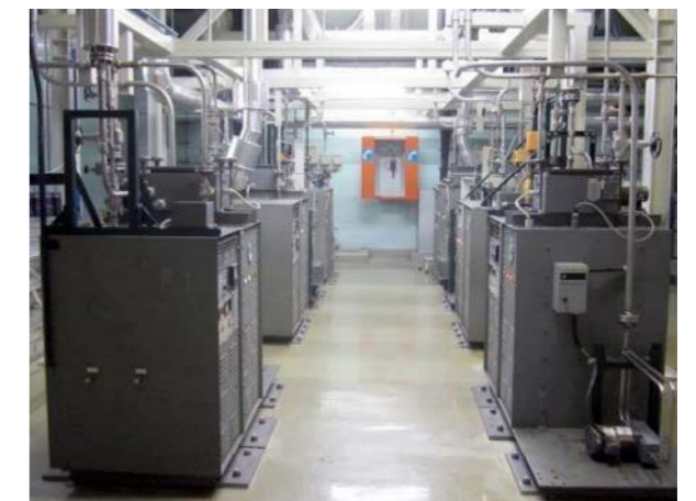
Equipment for the permanent monitoring of gaseous discharges at the Tihange nuclear power plant
